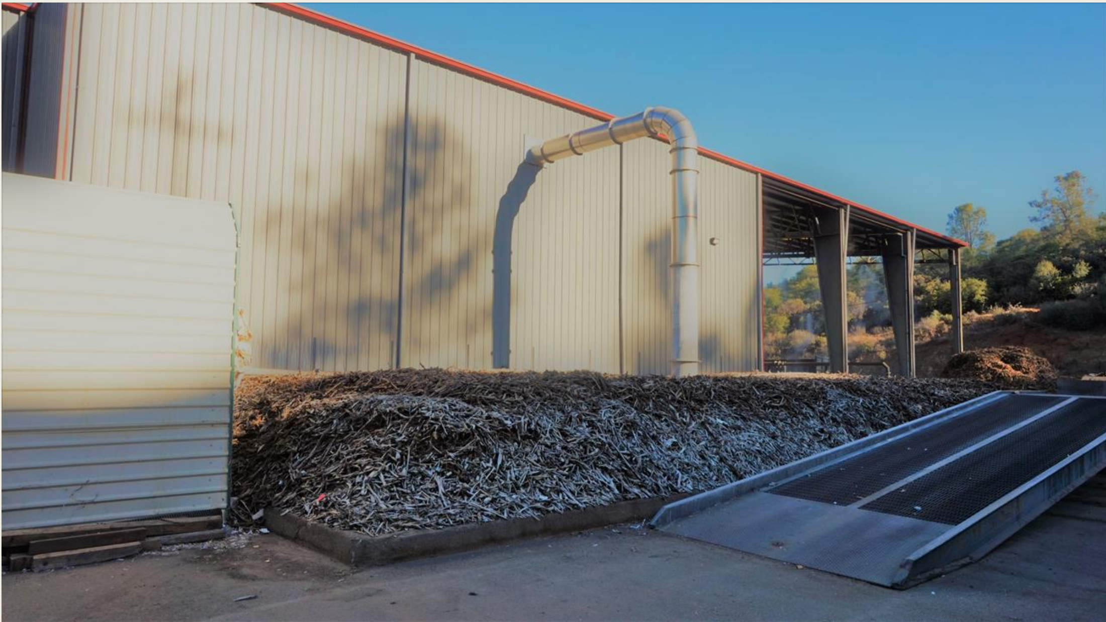
Biofiltration of the air to scrub odors
