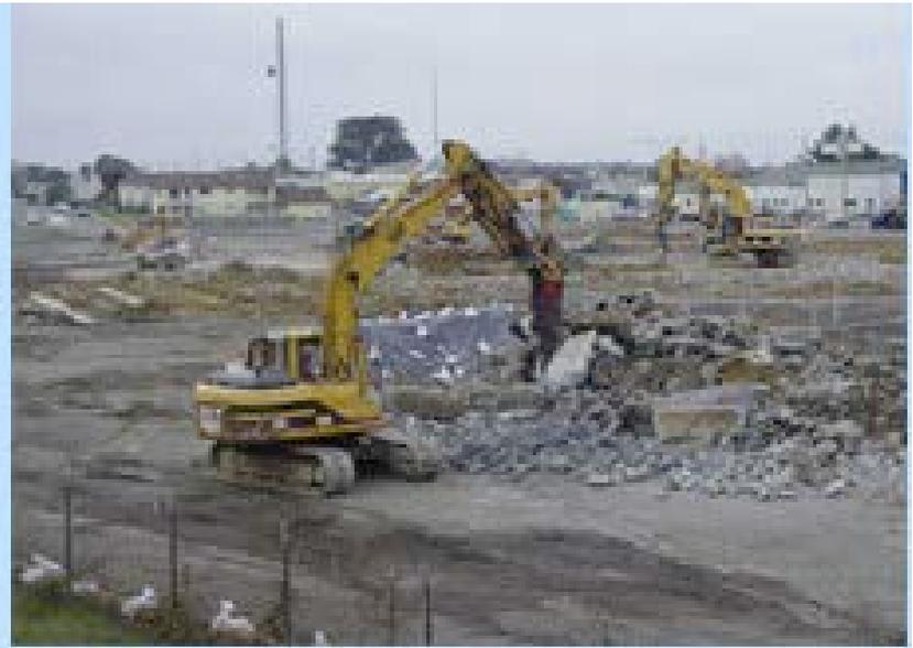
**Kernen Construction produces and sells recycled aggregate base. They take concrete, asphalt, bricks, glass and ceramics (toilets, sinks, etc.) and crush them for aggregate base. The products meet all specification for Caltrans class 2 aggregate base.**
