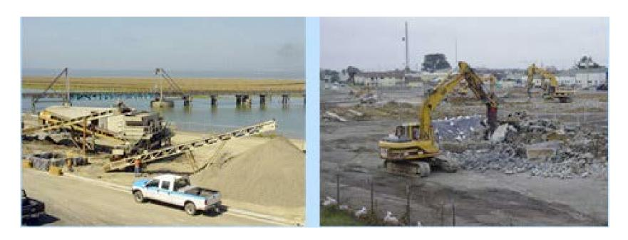
Kernen Construction produces and sells recycled aggregate base. They take concrete, asphalt, bricks, glass and ceramics (toilets, sinks, etc.) and crush them for aggregate base. The products meet all specification for Caltrans class 2 aggregate base.
